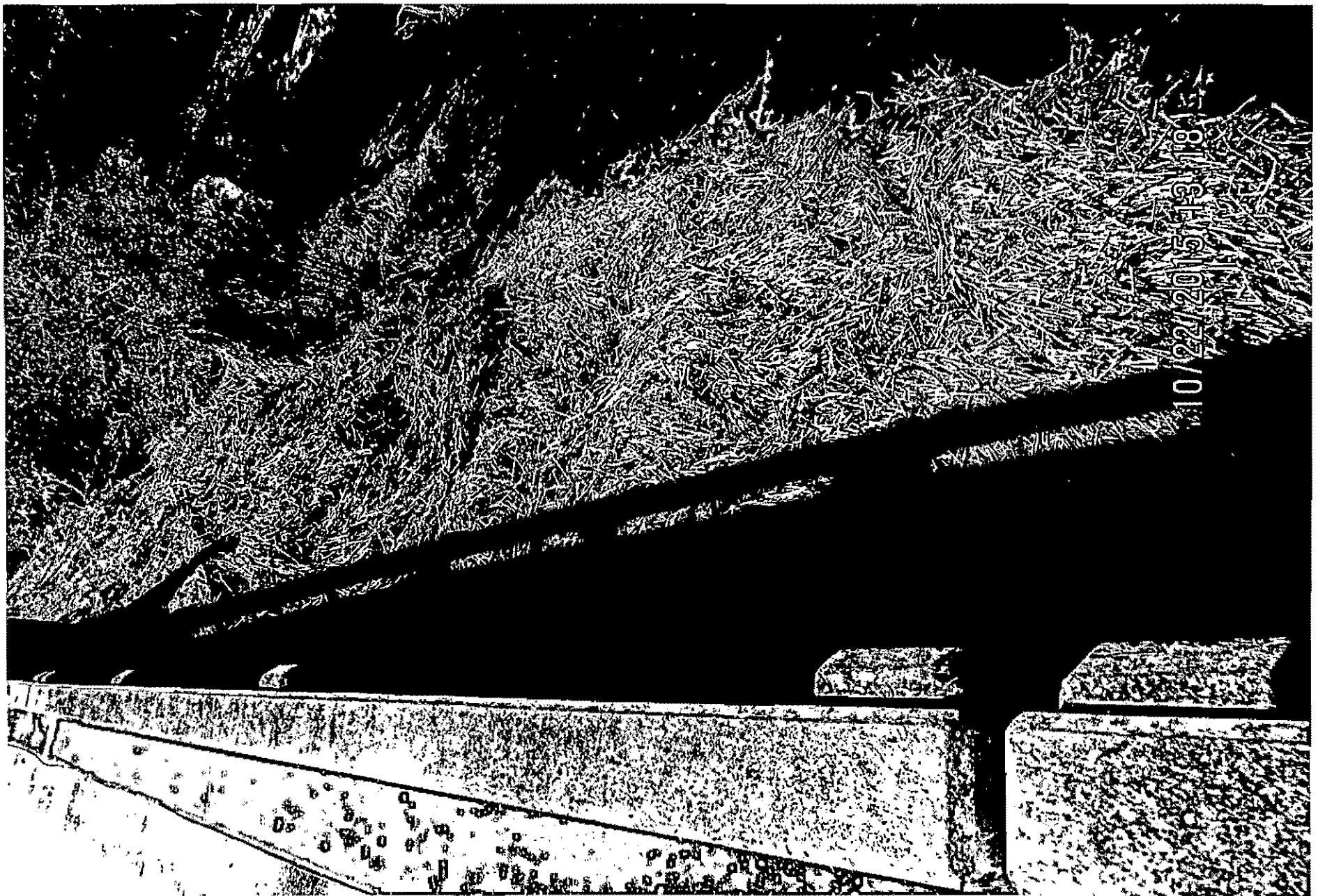
14-2-00301-0-12-00 2015 Debris Buildup Upstream Side of Span #1
