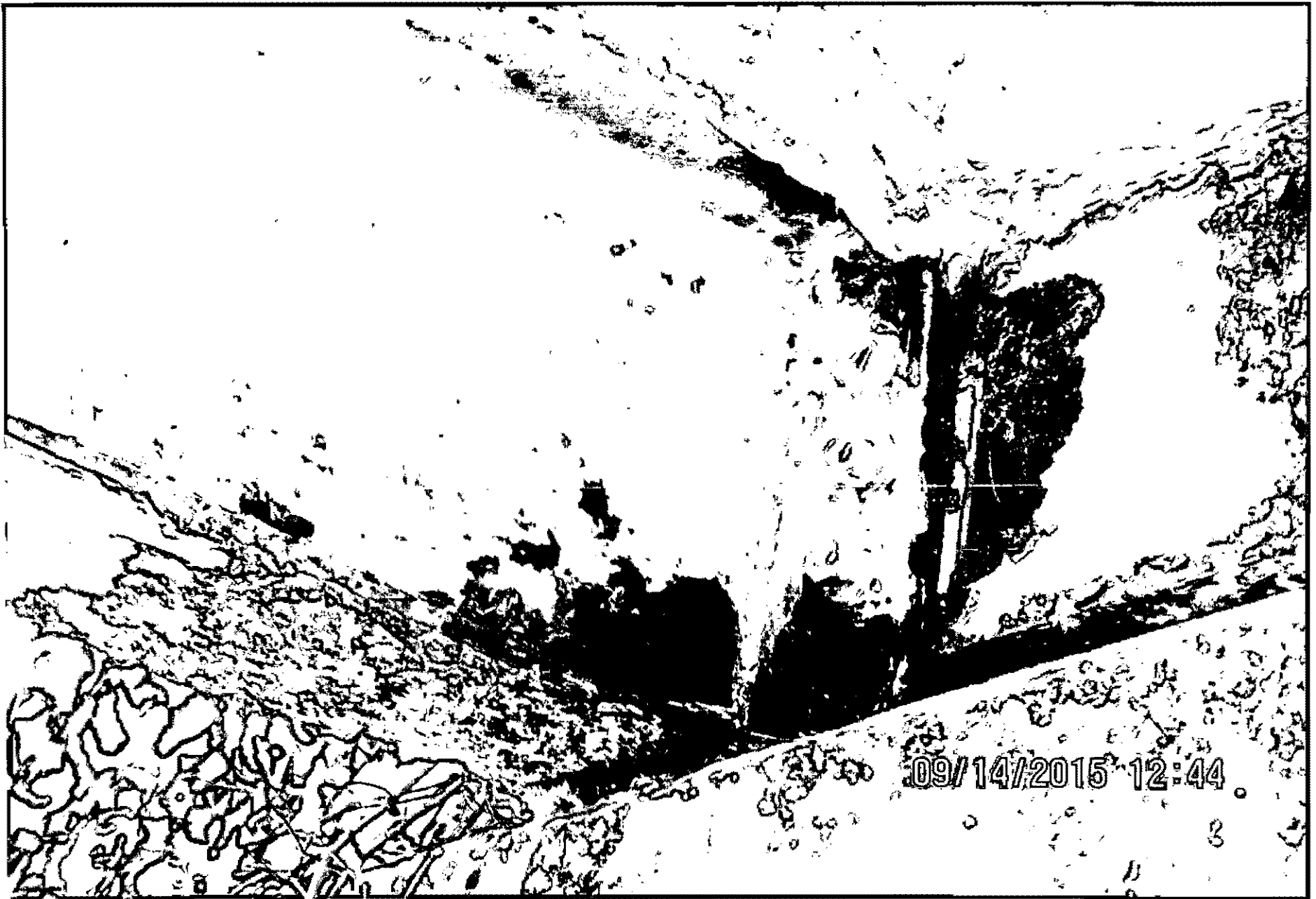
14-2-00301-0-12-00 2015 Beam 8 on Bent 15 Complete Section Loss on Diaphragms & Major Section Loss on Beam Ends
